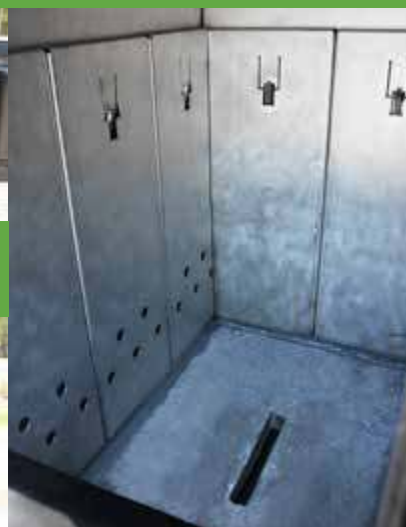
Air Panels & Gasification Manifold
